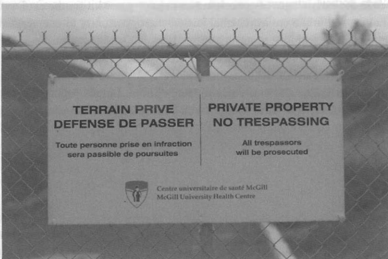
Figure 9.7 McGill University multi-billion dollar hospital complex under construction between working-class Saint-Henri and affluent Westmount.
