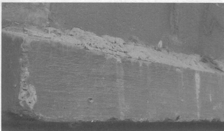
Figure 9.9 Air pollution on window ledge of highway-adjacent building in Saint-Henri.
